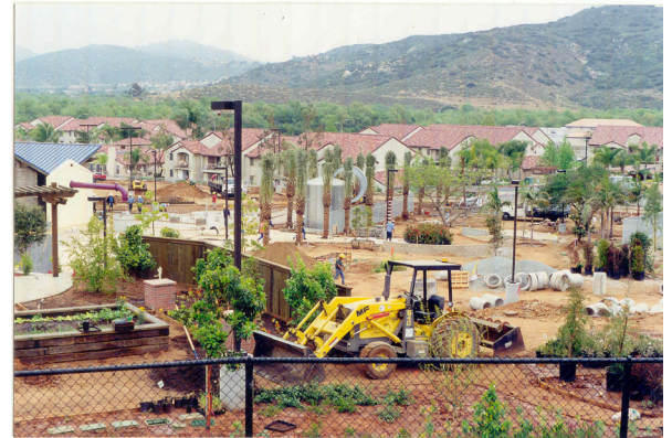
The Garden under construction, 1999
