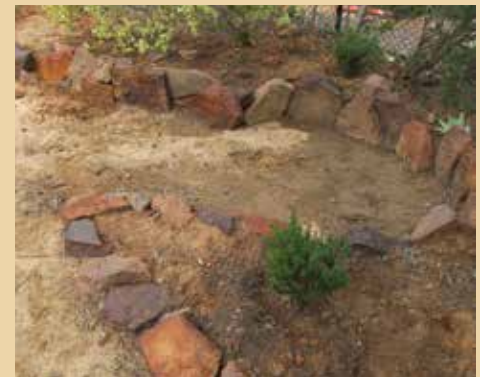
Urbanite Swale After Completion
